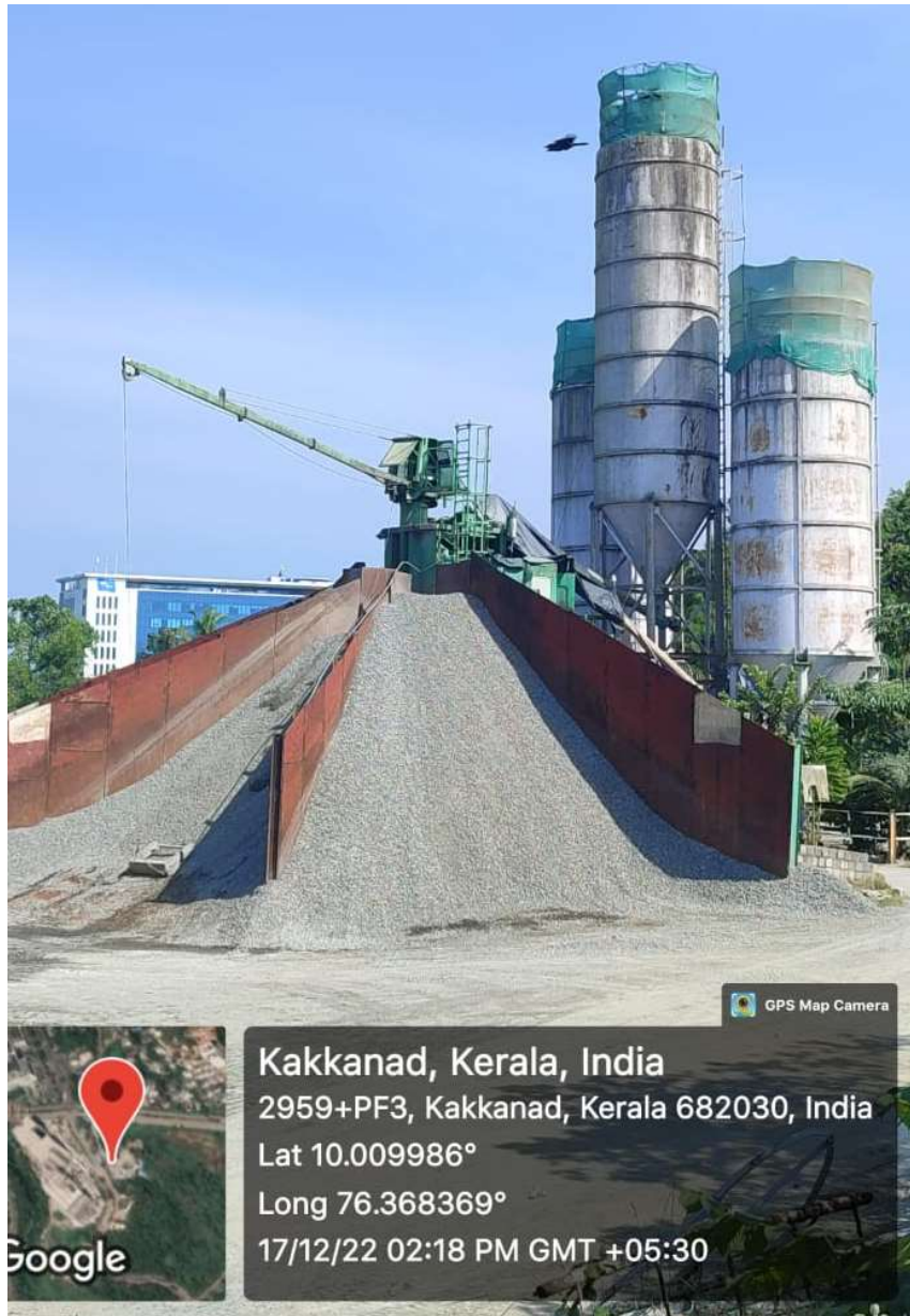
Ready mixed unit
