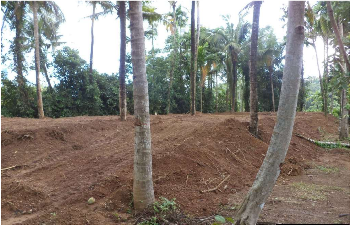
Top soil stacked in project site
