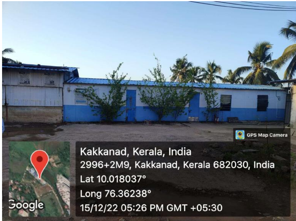
Facilities for labours
