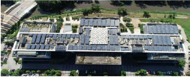
Rooftop Solar & Greenery
