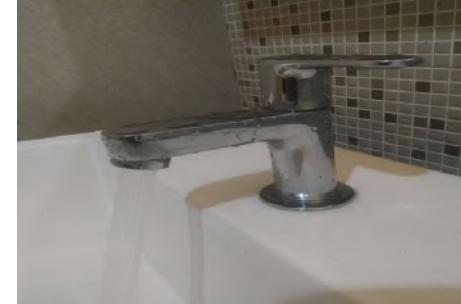
Discharge through 4 LPM Shower flow aerator
